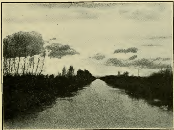
Brawley main canal supplying a large portion of Imperial Valley.
