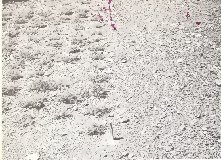
Figure 2.—The "lime line" is clearly visible on this graded coal-breaker refuse. The area on the left was limed; it produced a good cover of crownvetch. The area on the right was not limed; here no crownvetch survived.
