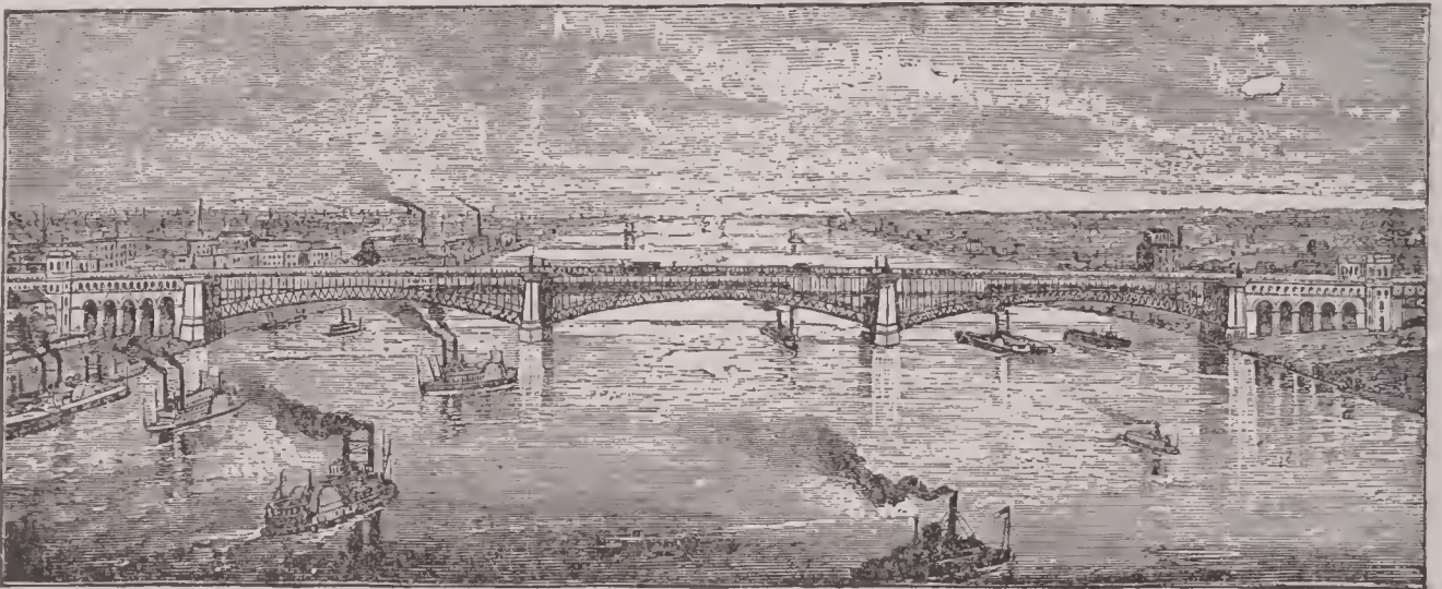
THE ST. LOUIS BRIDGE.
