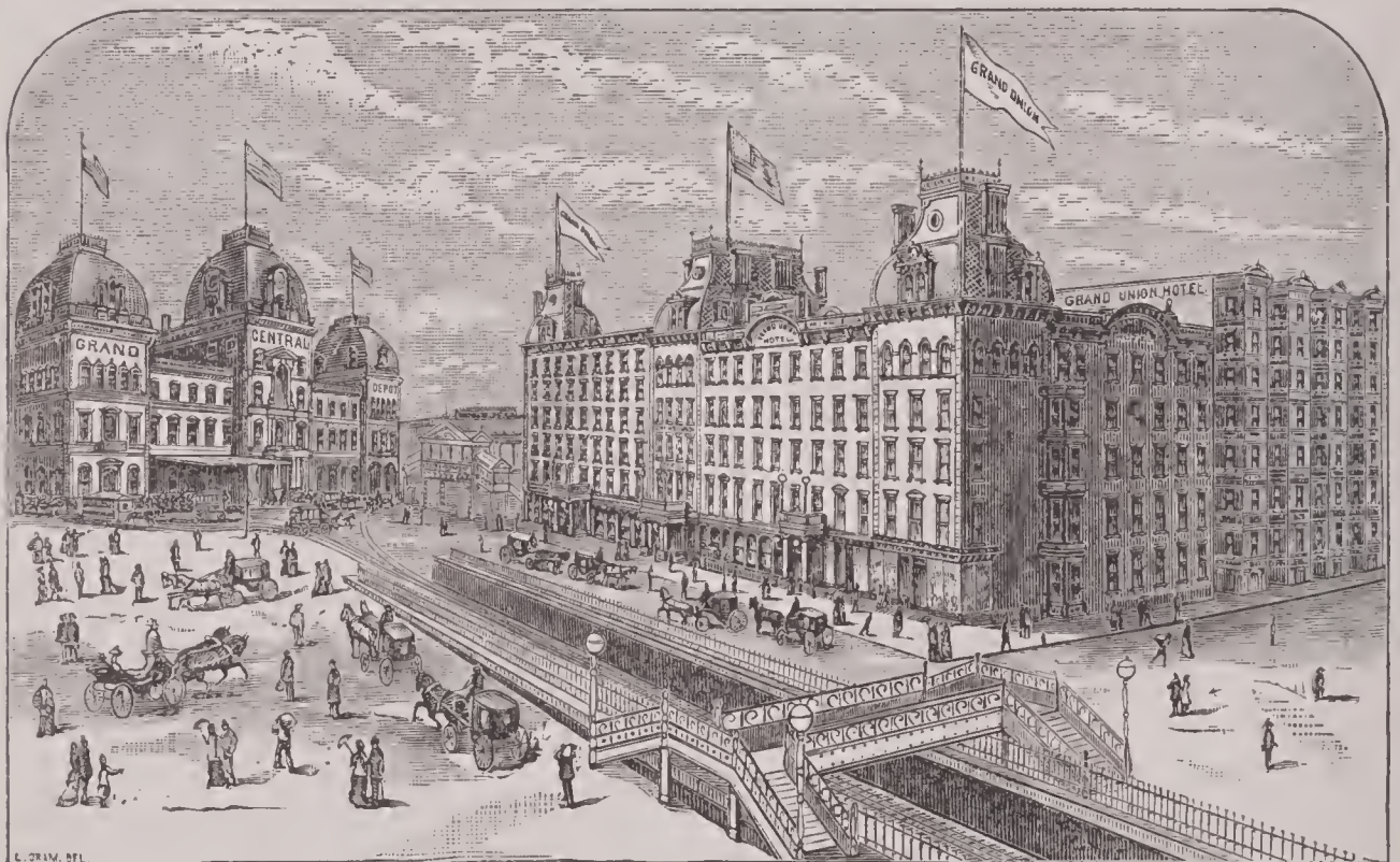
GRAND CENTRAL DEPOT—GRAND UNION HOTEL, FORTY-SECOND ST. AND PARK AVENUE.
