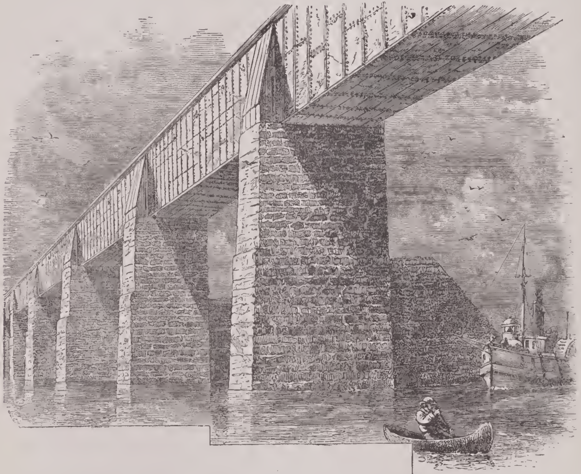
SECTION OF THE VICTORIA BRIDGE.
